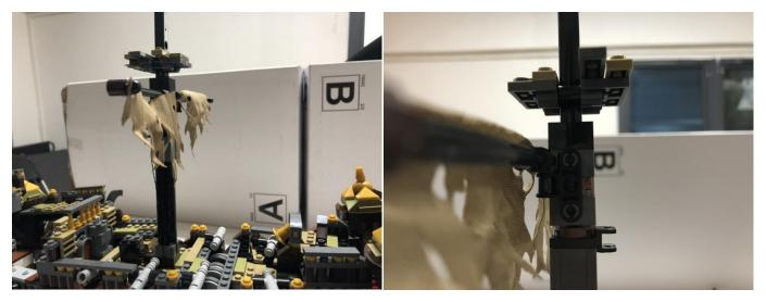
29) take a 30cm connecting cable, a warm white strip light. Connect the cable to one port on the strip light
